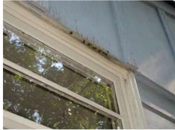
Honey bees are coming and going through a crack where the window casement meets the siding. Is that where the nest is? Nope! It is five feet to the left.
